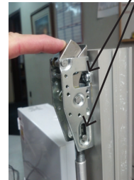
Top latch fully extended and deadlatched.
