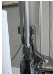
Top latch fully extended and deadlatched. Rod fully extended and flush with bell crank.
